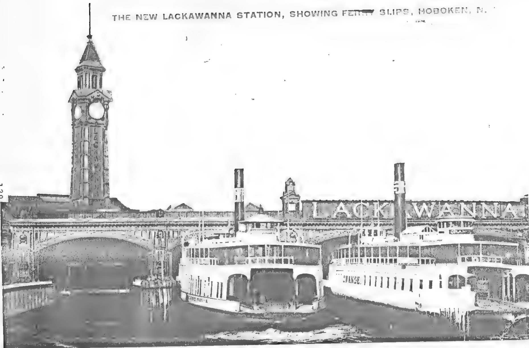
Enlargement of a postcard image of the terminal's river facade, showing Clocktower and ferries in the slips. Courtesy, Hudson City Historical Society, Theodore Conrad Collection.
